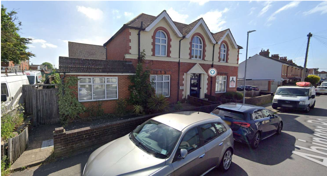
Existing front elevation viewed from Abinger Road
