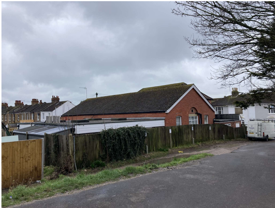
View towards the rear of the site from the north
